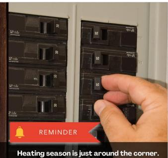
Heating season is just around the corner. If you have a heat meter, you can start getting heat credit with your October reading. Be sure the breaker to the heat meter is on. We encourage you to leave these breakers on year-round. Without power, the automatic meter reading can't detect trouble or report readings.
