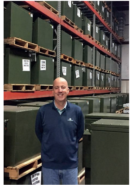
Matt Brandrup, president and CEO of Rural Electric Supply Cooperative (RESCO), stands in front of ERMCO three-phase transformers and single-phase padmount transformers. Photo courtesy of RESCO.
